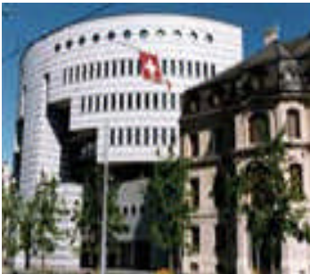
Botta 1 Building, Basel
