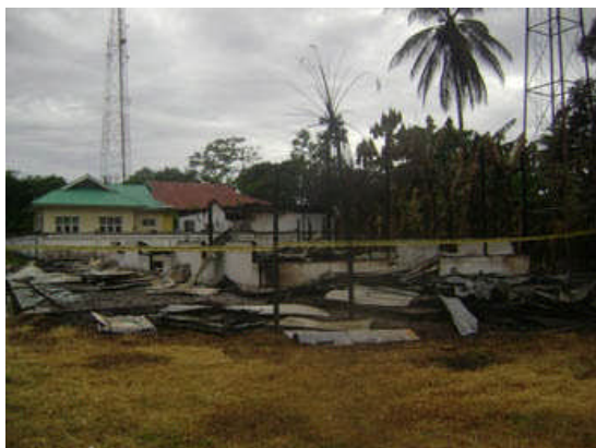
Destroyed building in Letwaru
